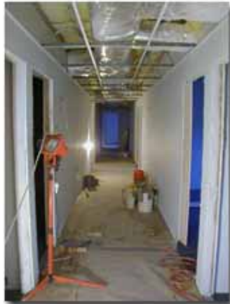
Building Catching Up
