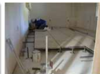
Access Floor installed
